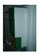
Normally the door is locked with a TVR1 door lock or a bar magnet, connected to the TT1 control terminal. In an emergency the door can be unlocked by pressing the integrated Emergency-Open switch. This will automatically set off the alarm siren and furthermore the yellow LED is switched on. The same applies if somebody tries to manipulate the TT control terminal (sabotage contact).
